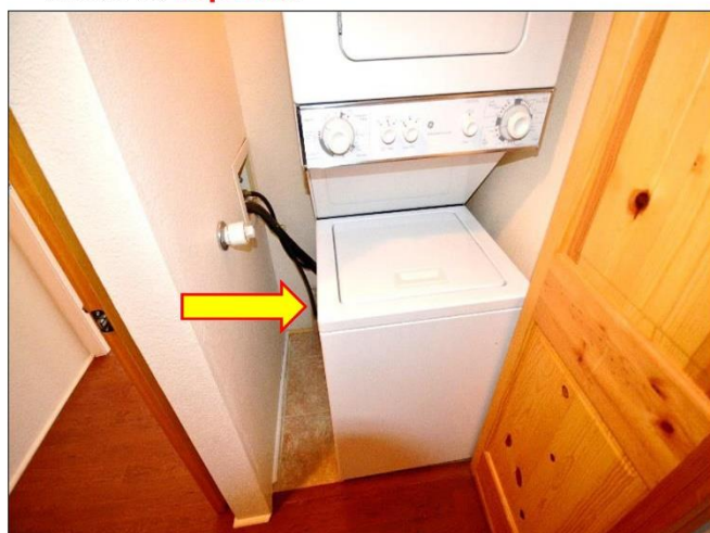
10. GE stacked Laundry washer & dryer's washing cycles are running squeaky and the washing machine will possibly need a new belt.
