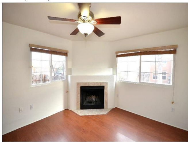
12. Living Room's Kiva Fireplace/ Ceiling Fan/ Pergo wood veneer flooring and the vinyl windows are in Satisfactory Condition .
