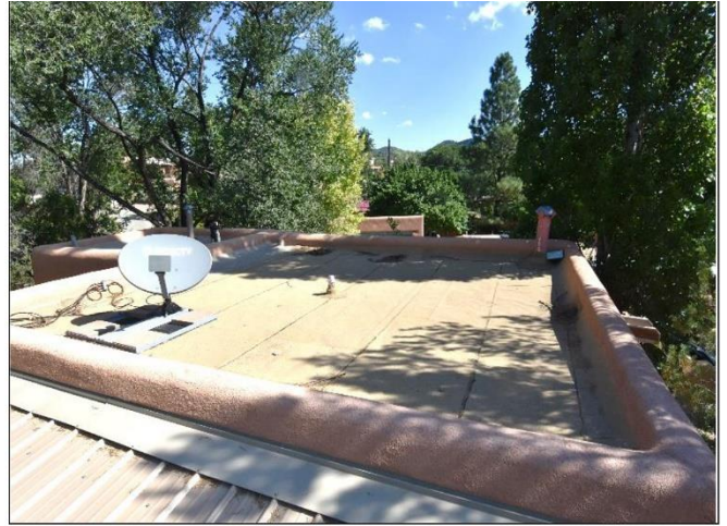
2. Propanel pitched roof attachment to parapets is in Satisfactory Condition.
