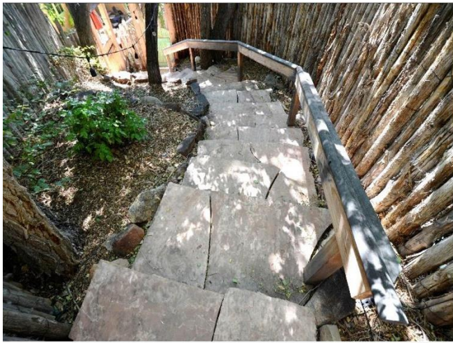
9. Flagstone stairs from the upper garden area is in Satisfactory Condition.
