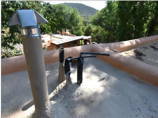
3. Small upper spray foam roof is in Satisfactory Condition.
