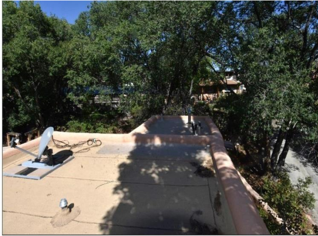
1. Torch-down roof membrane on the upper roof is in Satisfactory Condition.
