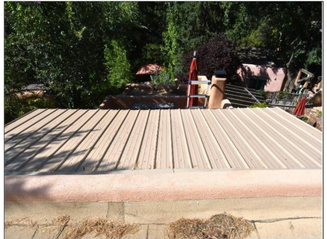
4. Propanel pitched roof over lower rooms is in Satisfactory Condition.
