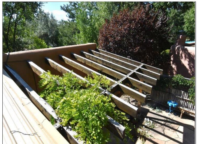
6. Exposed massive beams will need to be oil-sealed at least every 5-years.
