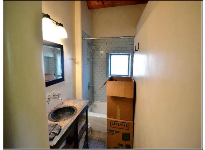
26. Downstairs bathroom with ceramic tile floors, Kohler bathtub and custom metal sink are in Satisfactory Condition.
