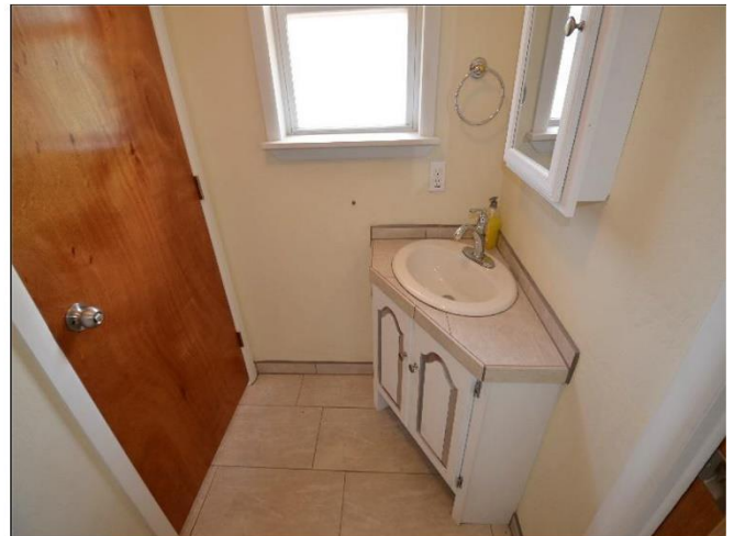
40. 2nd Floor, (Main Floor) Master Suite Bathroom with corner Vanity is in 3/4 Bathroom is in Satisfactory Condition.
