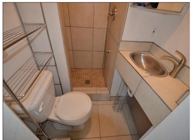
42. 3/4 Basement Bathroom is in Satisfactory Condition.
