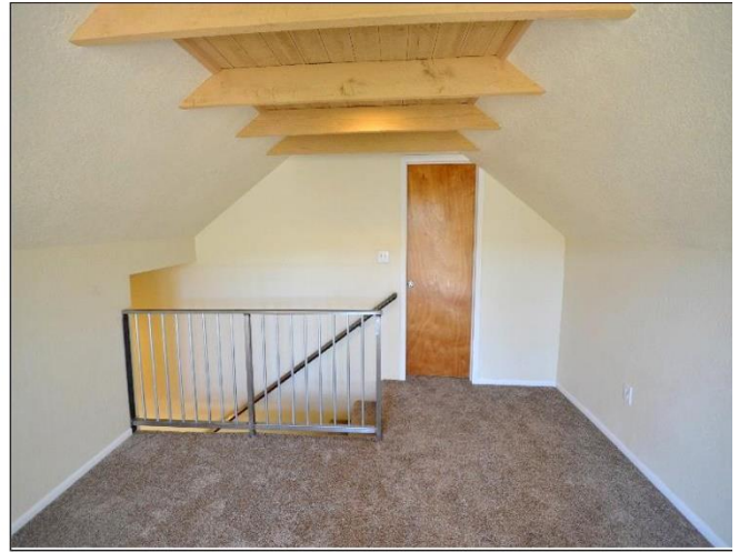
26. 3rd floor landing with hand railing is in Satisfactory Condition
