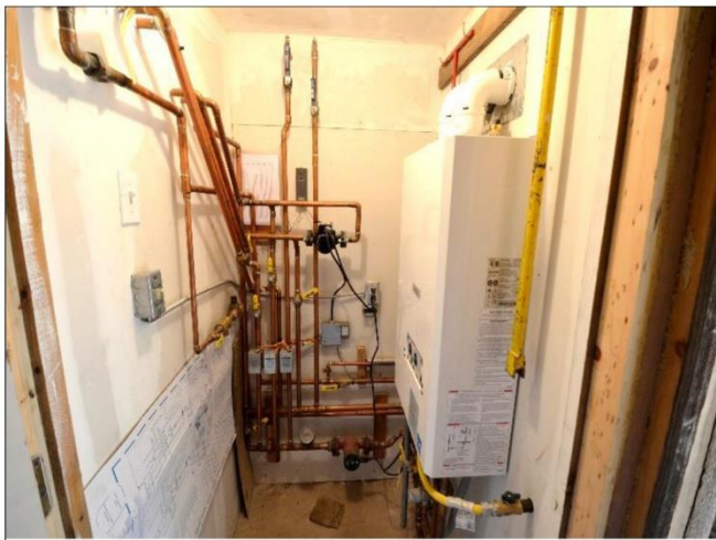
9. Mechanical closet setup for domestic and radiant heating by using Propane fuel
